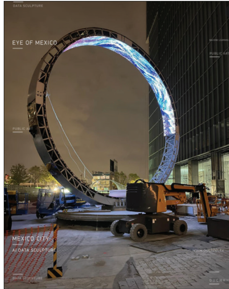
Progress images of the Eye of Mexico installation.
