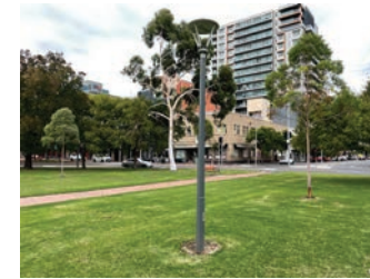
EXISTING LIGHT POLES
